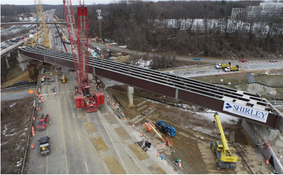
The girders measure 11 feet tall with the longest spanning 295 feet and the heaviest pieces erected weighing over 80 tons.
