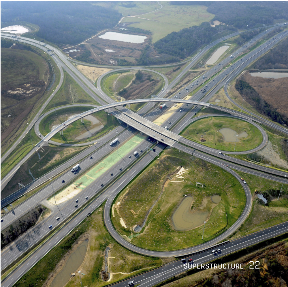
Below: The Intercounty Connector, Contract C for the Maryland Department of Transportation State Highway Administration included 23 new bridges and required the movement of over 2.6 million cubic yards of earthwork.
